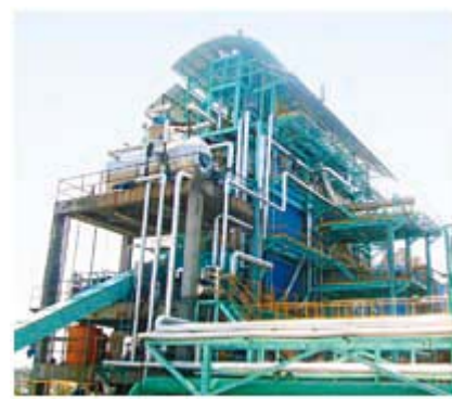
Wood biomass power generation facility which began operation in March 2008
