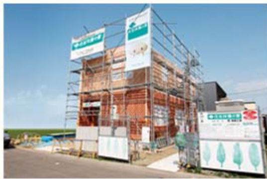
The residence under construction
