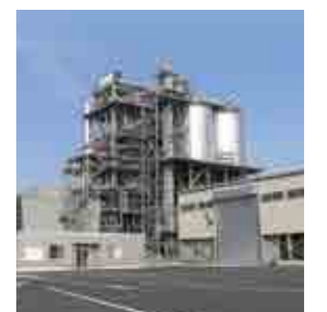
Exterior view of the Kawasaki Biomass Power Plant
