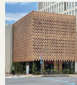
This building also contributes to local production for local consumption by cedar from the Tama area for the exterior
