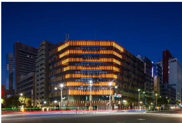
External renovation of office building
