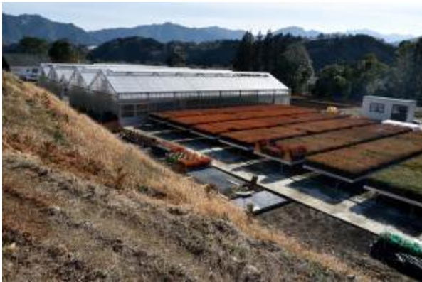
Image of completed first-stage development (Togo Tree Breeding Center, Hyuga Forestry Office)
