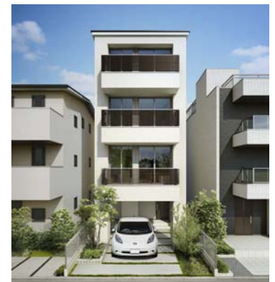
Exterior view of the BF-Fireproof (four-story)
