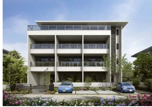
Forest Maison BF-Fireproof (four-story owner-occupied rental units)
