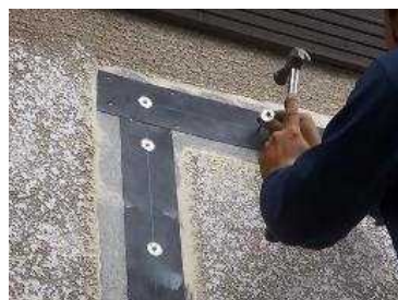
Photo left: Attaching of base sheets and hammering in of washer-attached nails.
