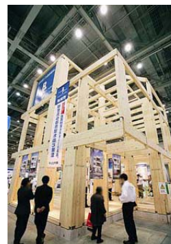
Full-size actual structure using the Big-Frame construction method
