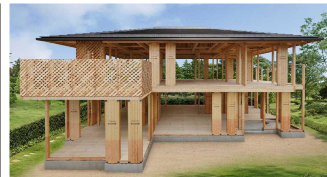
Big-Frame Construction Method
