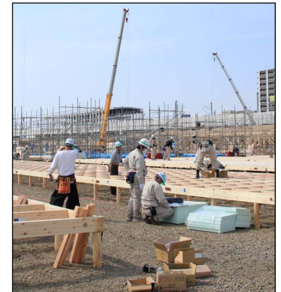
Construction of emergency housing (Miyagi Prefecture)
