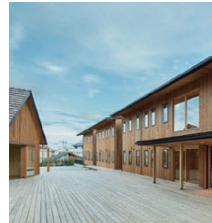
Annex at Senri Rehabilitation Hospital
