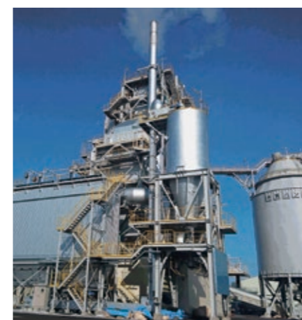
Hachinohe Biomass Power Plant
