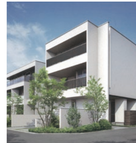
Forest Maison apartment housing (exterior)
