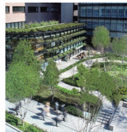
Environmental landscaping (Mitsui Sumitomo Insurance Surugadai Bldg. with adjacent "ECOM (eco + communication)" space)
