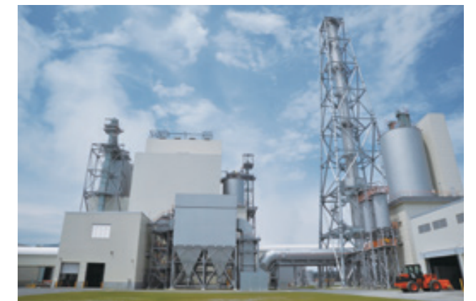
Mombetsu Biomass Power Plant
