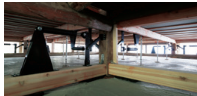
Sumitomo Forestry Group's original energy-absorbing dampers reduce the amount of shaking experienced by buildings during earthquakes
