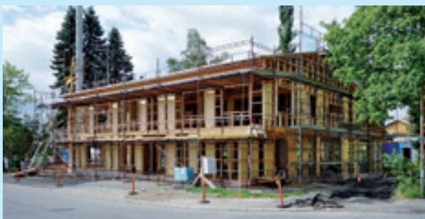
Student dormitory being constructed using our BF configuration.
