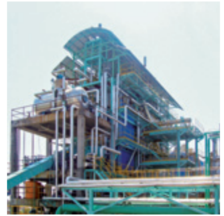
The wooden-biomass boiler at RPI, our building materials manufacturing facility in Indonesia.
