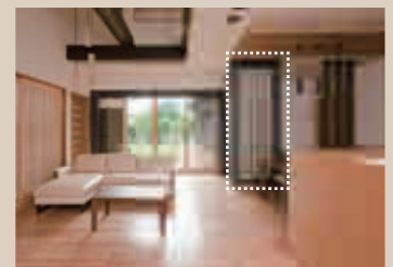
Glass block shear wall
