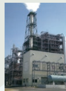
Kawasaki Biomass Power Plant
