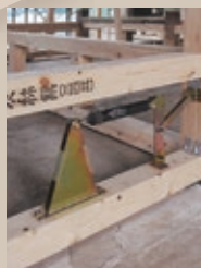
Sumirin CEM Construction Method
