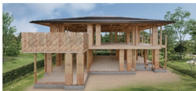
Structural framework of Big-Frame construction method
