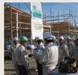
President Akira Ichikawa (in green helmet) visited 15 sites in the disaster region, including the temporary housing construction site, to see conditions for himself and supervise activities.
