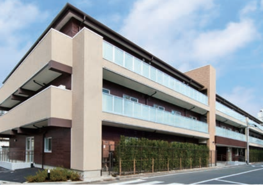
Three-story fire-resistant elderly care facility
