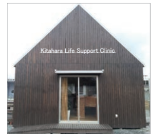
A health clinic built using MOCCA HUT temporary construction in Higashimatsushima City
