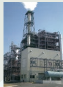
Kawasaki Biomass Power Plant
