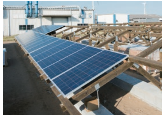
Environment-friendly wooden frames for solar panels
