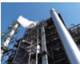
Kawasaki biomass power plant
