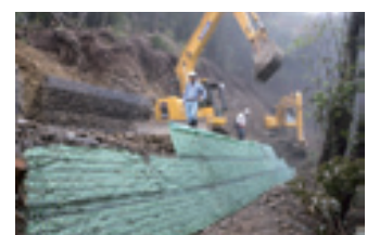
Developing a forest road along steeply inclined land
