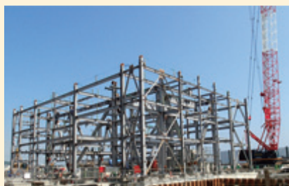
Construction under way in Mombetsu, Hokkaido
