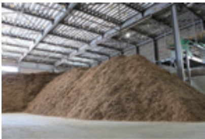
Chip yard built next to the biomass power plant
