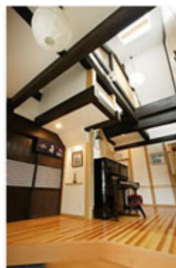
The previously concealed crossbeam is exposed under in the vaulted ceiling in the bright entrance hall
