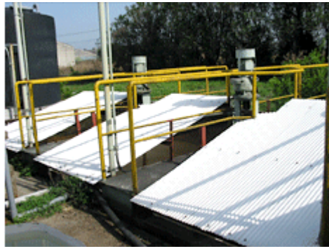
A roof was built over a storage pool of effluent and raw water to prevent rain from entering.
