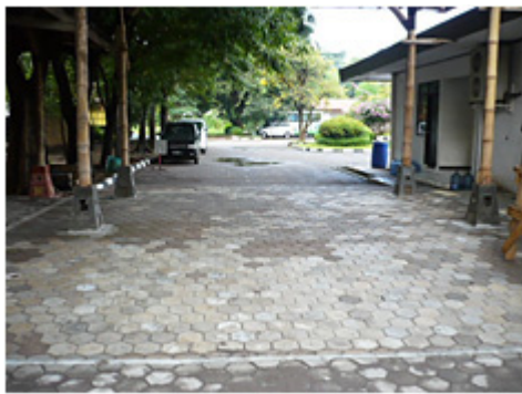
Example of construction work using RPI's roadbed materials
