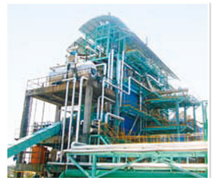
Wood biomass boiler
