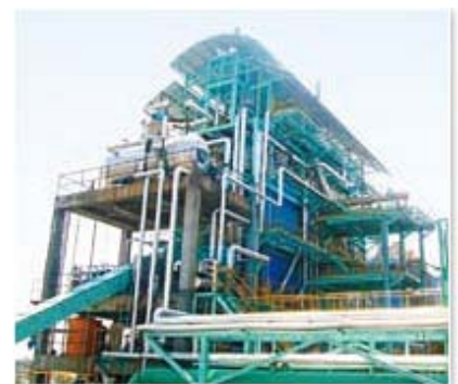
Wood Biomass Boiler
