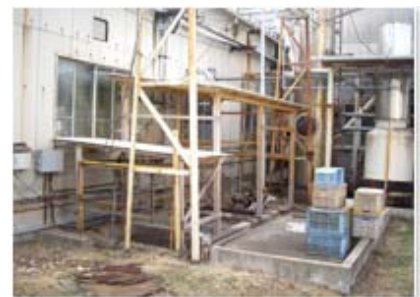
Roof Installation at No. 1 Plant
