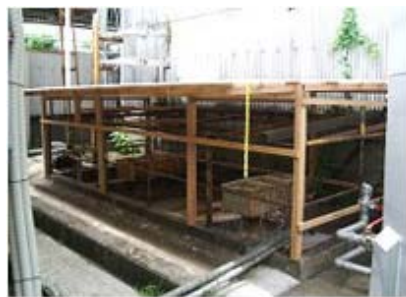
Roof Installation at No. 2 Plant Pit
