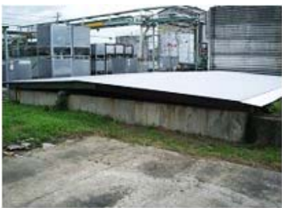
Roof covering treated water storage pool
