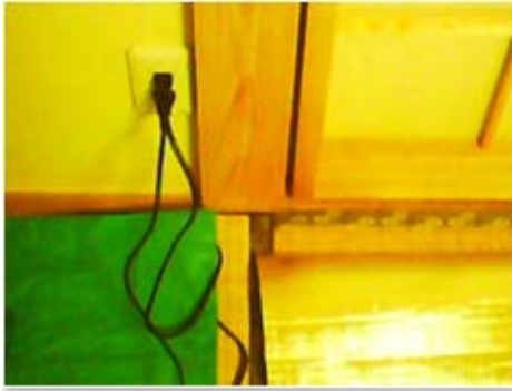
Small gaps that allow outside air in cannot be seen with the naked eye
