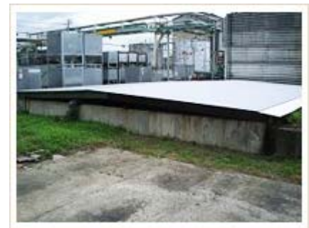
Roof covering treated water storage pool
