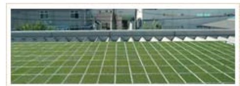
Installation of Moss Folded-Plate Roof Greening System
