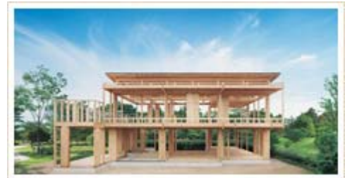
Home Using the Big-Frame Construction Method
