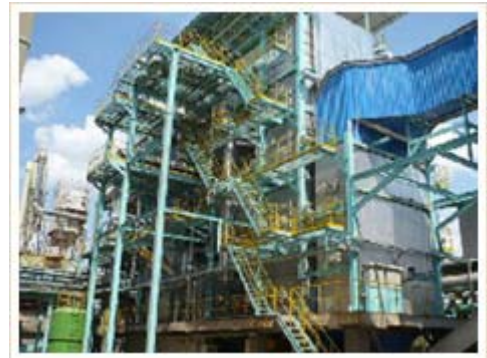
RPI's wood biomass boiler
