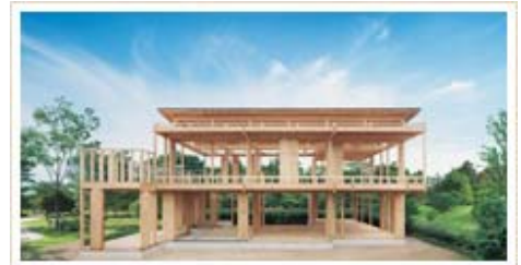
Home Using the Big-Frame Construction Method
