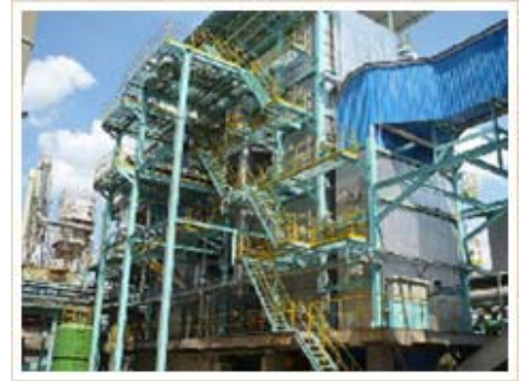
RPI's wood biomass boiler
