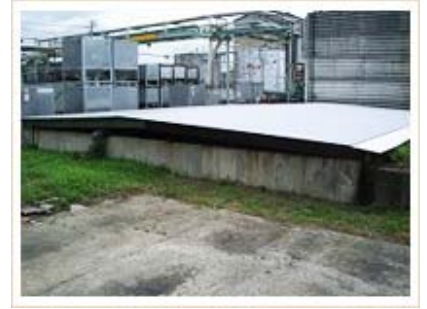
Roof covering treated water storage pool
