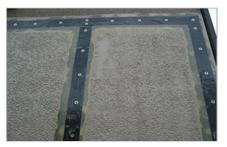
Seismic -Resistant Mortar Outer Wall Base Sheets Installed
