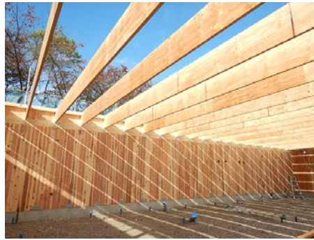
Wood CLT Convenience Store Construction
