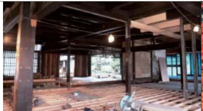
Remodeling work by Sumitomo Forestry Home Tech. Co., Ltd.
