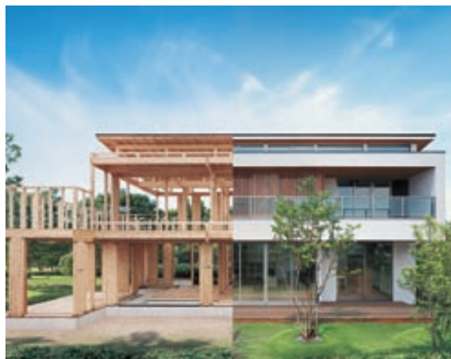
The BF-Si line of the Company's proprietary Big Frame construction method allows for an exceptionally high degree of layout flexibility including creation of large open spaces.
