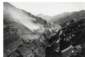
The Besshi Copper Mine was in a state of degradation during the Meiji era due to the effects of mining operations (stored among Sumitomo Historical Archives)
