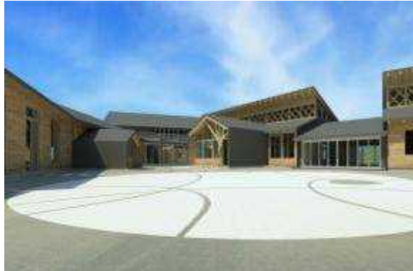
Elementary school disaster relief work (Miyagi Prefecture)
