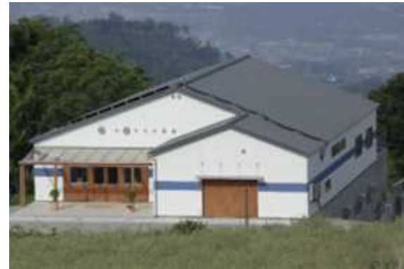
Winery (Nagano Prefecture)
