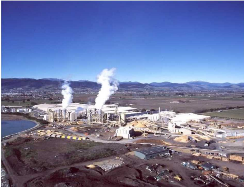
Nelson Pine Industries Ltd. MDF/LVL manufacturing plant
