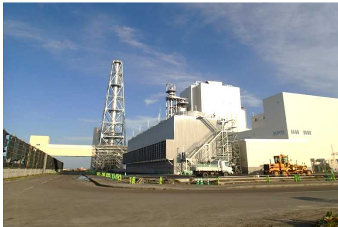
Mombetsu Biomass Power Plant Capacity: 50 MW (Enough to supply about 60,000 regular households)
