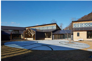
Miyanomori Elementary School in Higashimatsushima City
