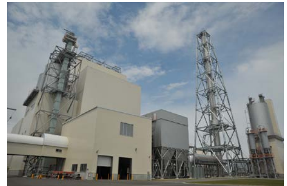
Mombetsu biomass power generation
