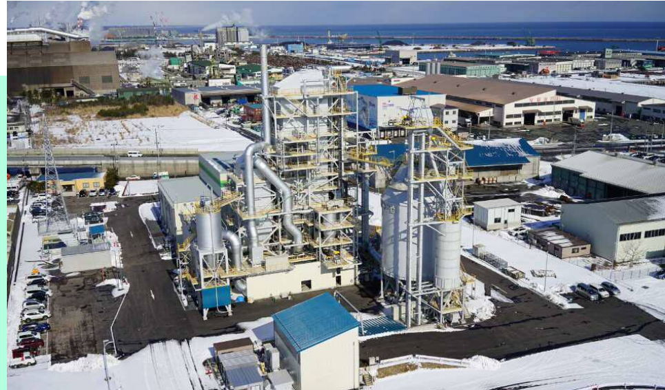
Hachinohe biomass power generation business started operation in April 2018
