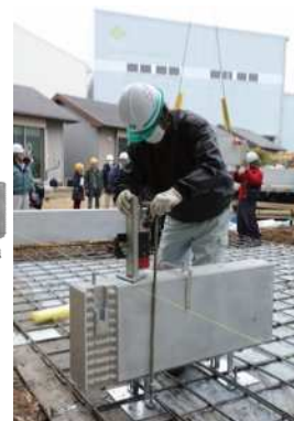
Pre-casting of foundations
