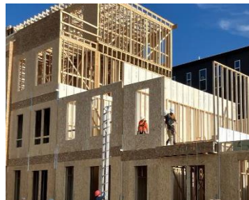
Wall panel construction
