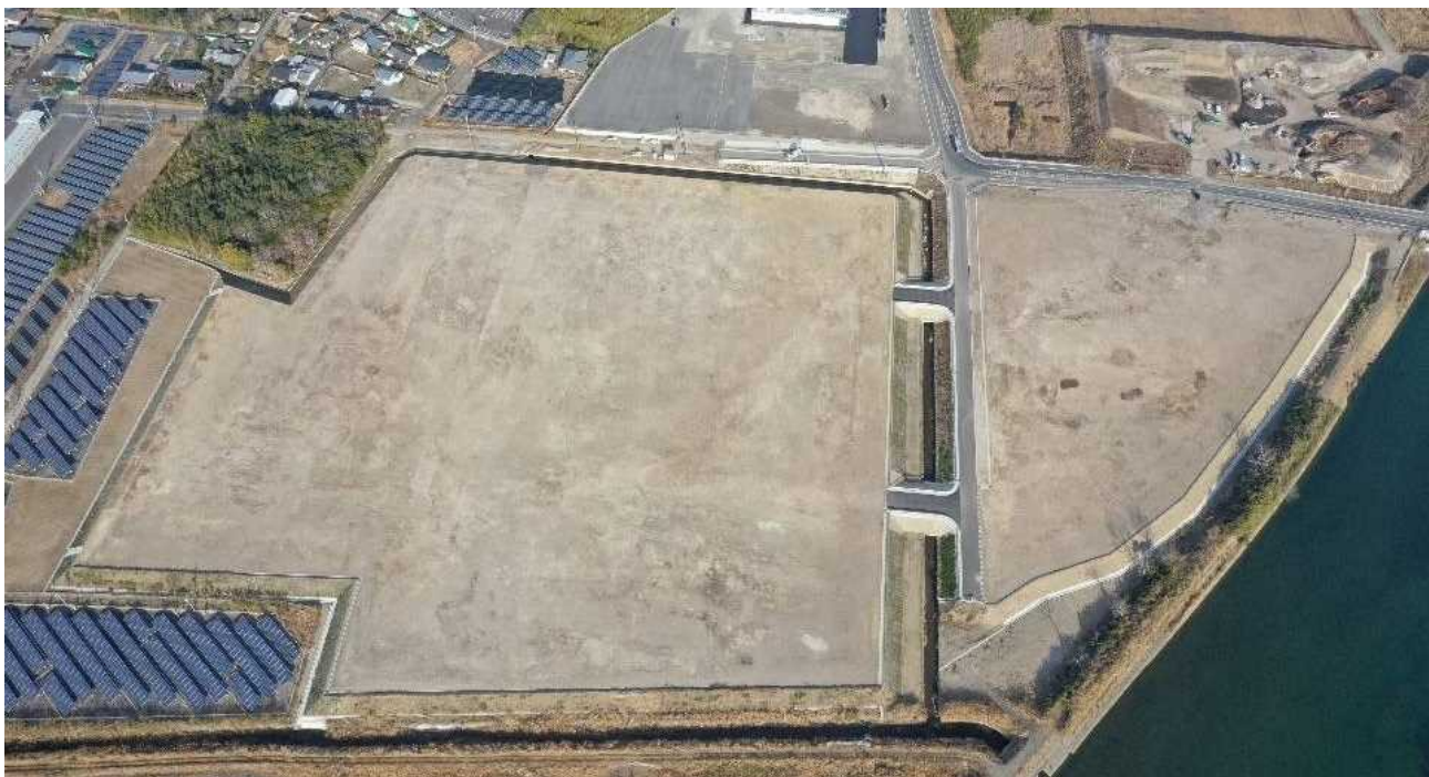
Aerial photograph of Shibushi City Seaside Industrial Park (Industrial Lot 5) [source: Shibushi City]
