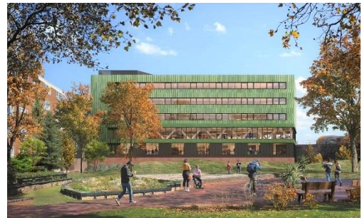
A 6-story mass timber office building in London currently under construction by Sumitomo Forestry and Bywater (image)
