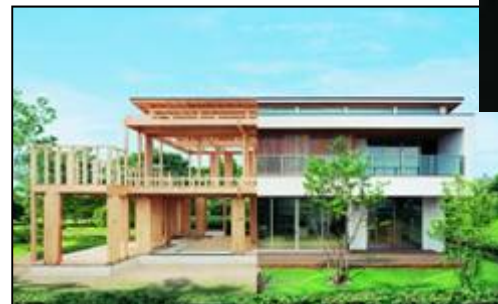
Big-Frame Construction Method
