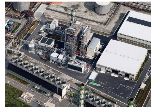
Kawasaki Biomass Power Plant
