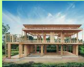
Quick to Introduce CAD / CAM and Precutting, Modernization of the Construction of Wooden Houses
