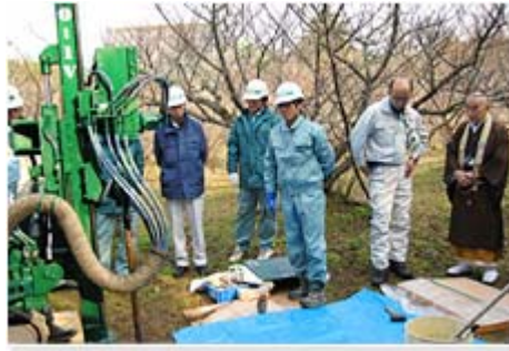
Omurozakura soil investigation
