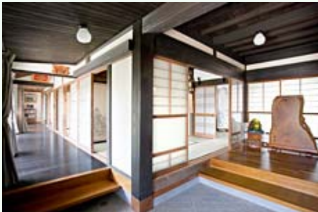
The left-hand entryway step uses Japanese zelkova wood from the original structure
