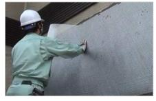
Earthquake-Resistant Mortar Outer Wall Net Temporary Fix
