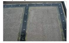
Earthquake-Resistant Mortar Outer Wall Base Sheets Installed
