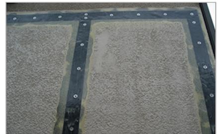
Seismic -Resistant Mortar Outer Wall Base Sheets Installed
