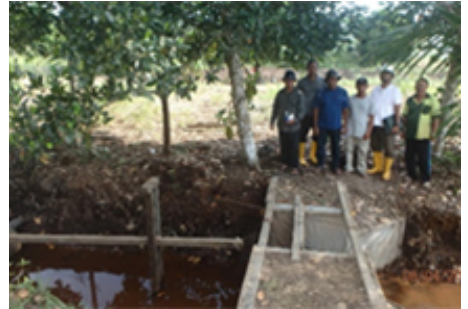
Ladakh Water Level Management Infrastructure
