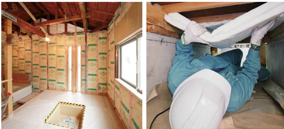
Installation of a Thermal Insulator
