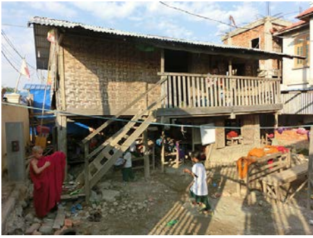
School before rebuilding
