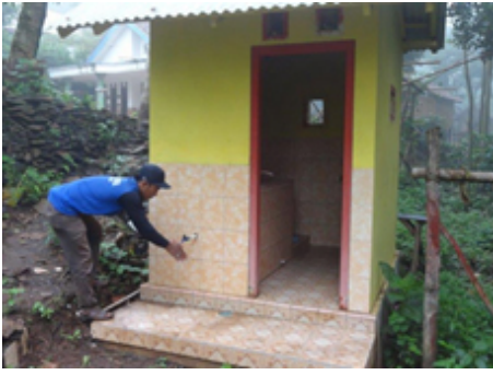
Public Bathrooms Set Up in Village
