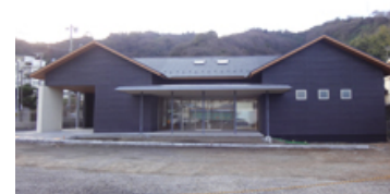
Exterior of new Sumirin Wood Peace Office Building
