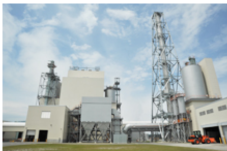
Mombetsu Biomass Power Plant
