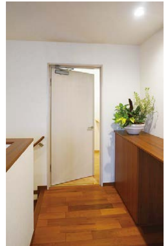
Own branded wooden fire-prevention doors made from balsa
