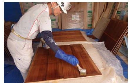
Cleaning drainage water stains
