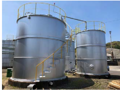
Biological processing facility (aeration tank)
