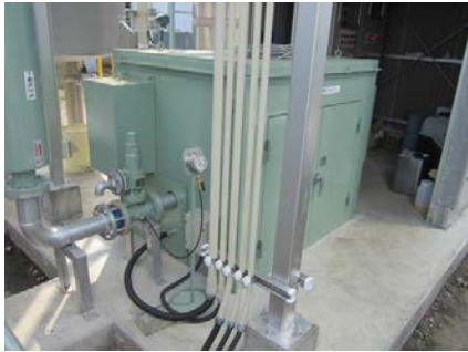
Biological processing facility (aeration blower)
