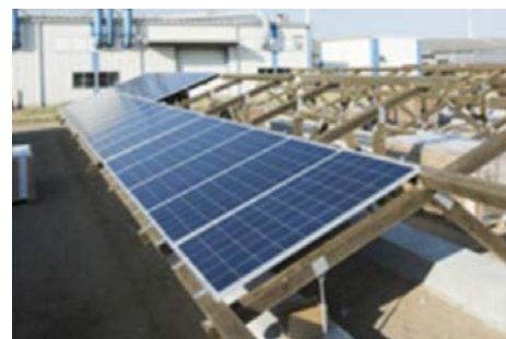
Solar panels and environmentally friendly wooden frames
