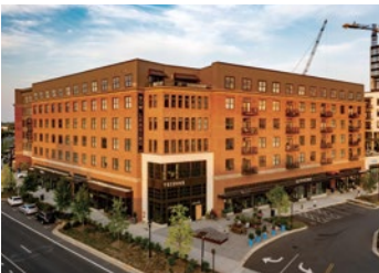
Atherton project: Wooden (wood-frame construction method) seven-floor multi-unit residential building (North Carolina, USA; sold in 2021)
