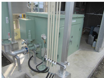
Biological processing facility (aeration blower)
