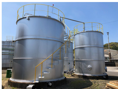
Biological processing facility (aeration tank)
