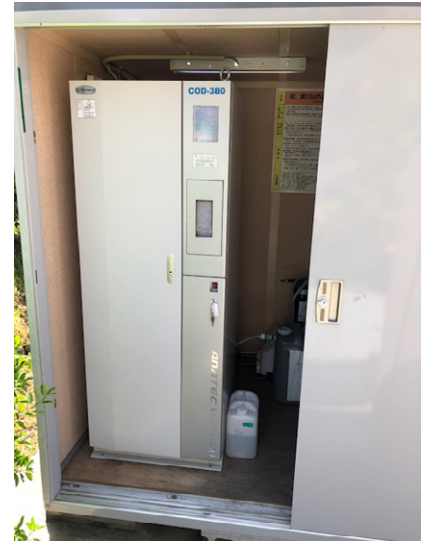
Measuring the COD of effluent
