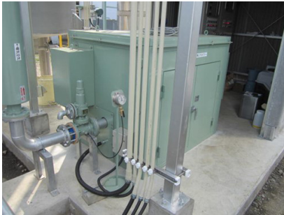
Biological processing facility (aeration blower)
