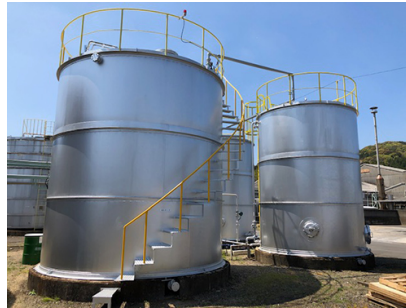
Biological processing facility (aeration tank)
