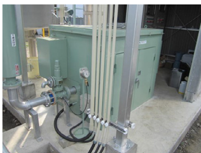
Biological processing facility (aeration blower)
