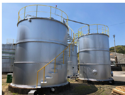
Biological processing facility (aeration tank)
